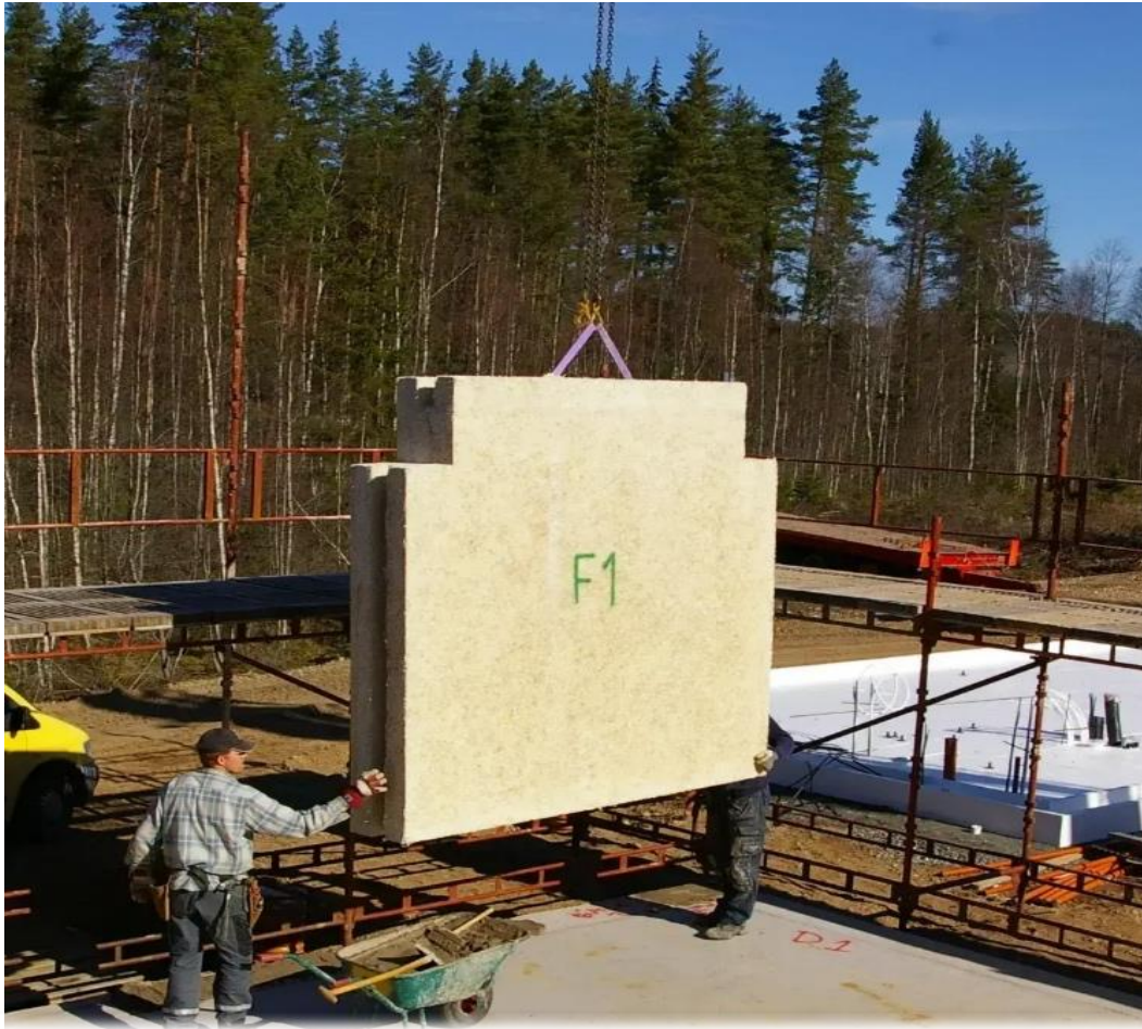
Step 3: Construct building using WWC – LWE systems
